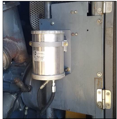
Picture 2 (After Installation)
