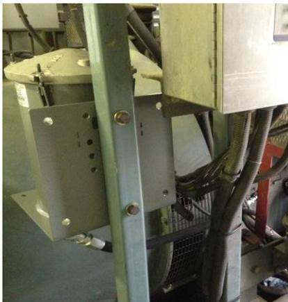
**Picture 3 (Mounting Method-MTU 16V2000)**
