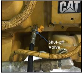
Picture 5: Shut-off valve & Supply hose connection
