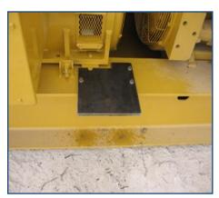
**Picture 4**: Mounting plate install.-Rail Mounted (Flat plate Set-up)
