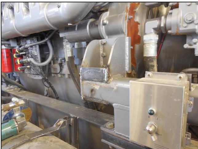
Picture 3: Reinforcement of mounting location
