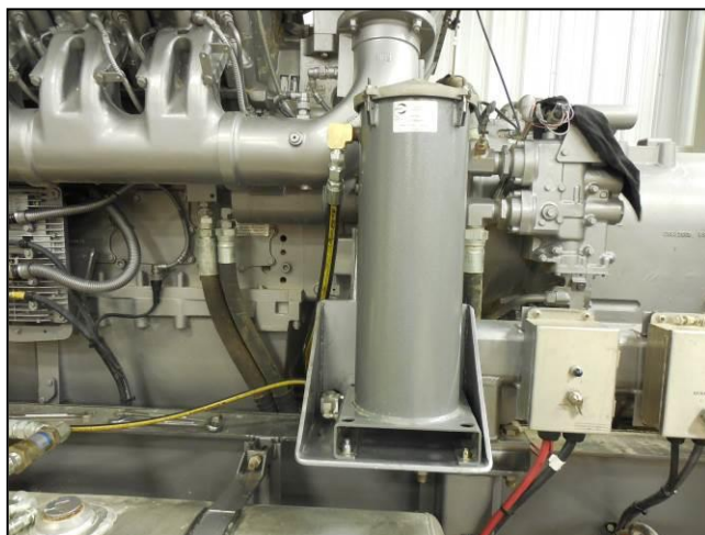
Picture 16: Return Hose Install & Orientation
