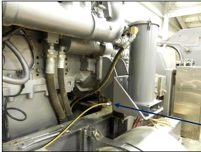
Picture 13: Installation of Supply Hose Assembly
