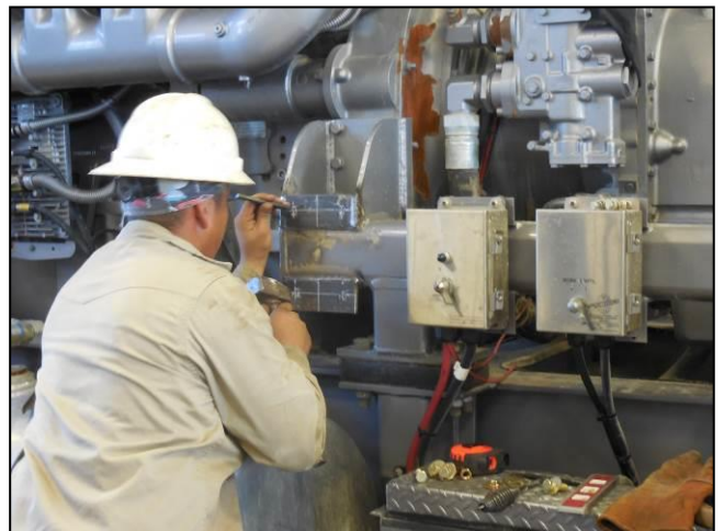
Picture 4: Marking of Hole Centers for Drilling
