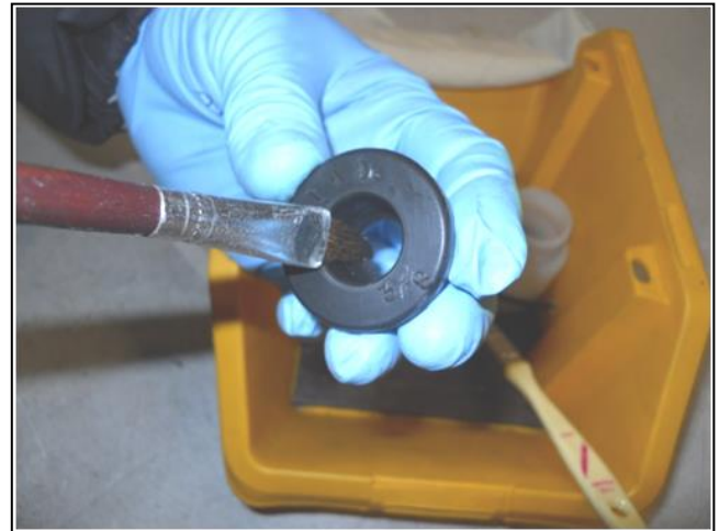
Picture 8: Grommet Prep/Installation
